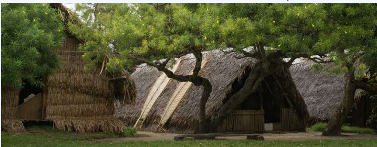
Traditional nakamal buildings, Vanuatu. maison-monde
